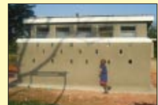
Latrines for the girls
