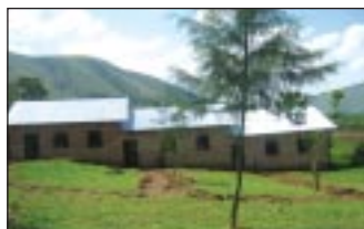
3 classroom block with roof 2009
